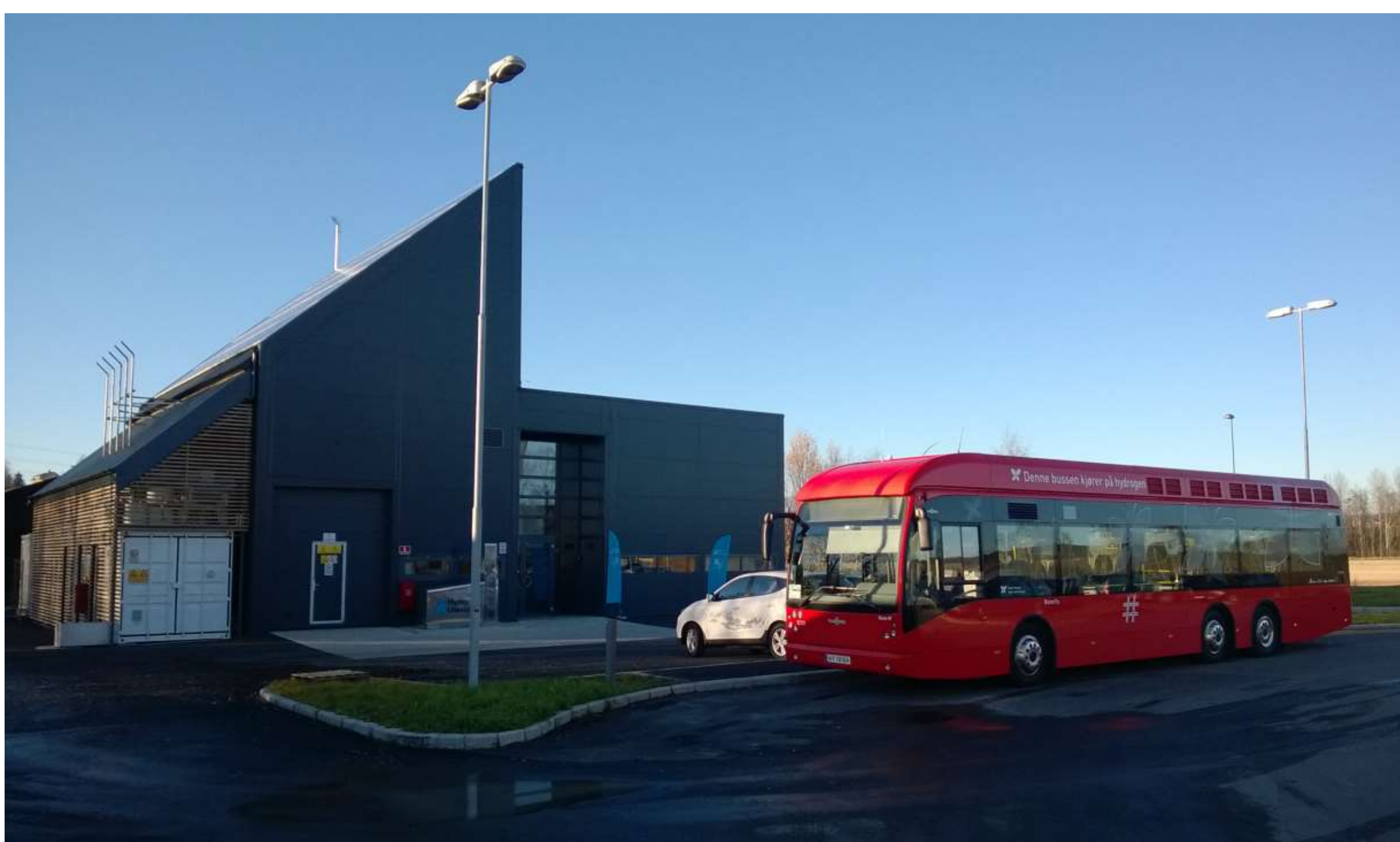
Water Electrolysis & Hydrogen Refueling
